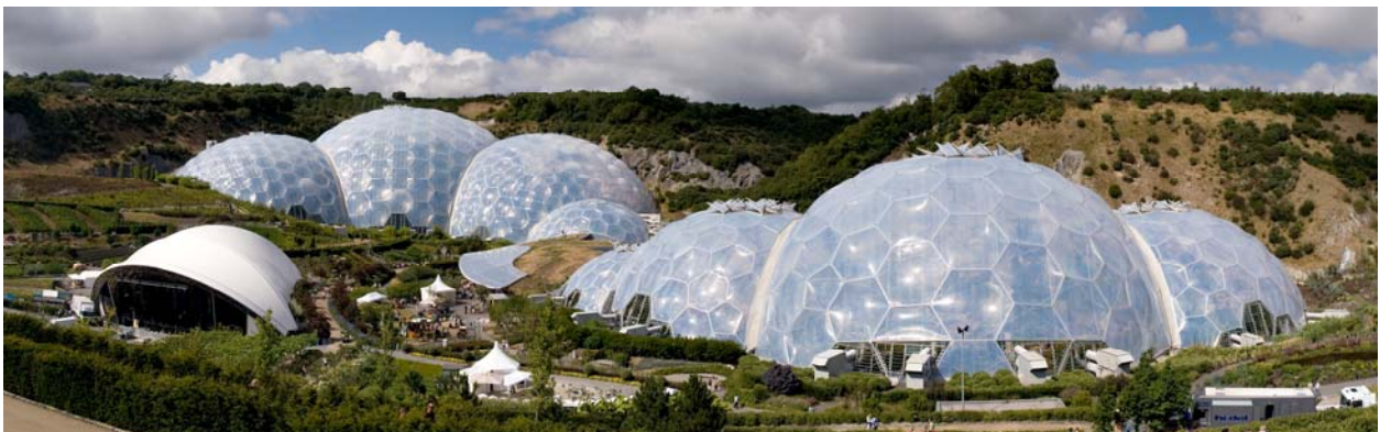
Eden Project geodesic dome environment, Cornwall, England, completed 2001
